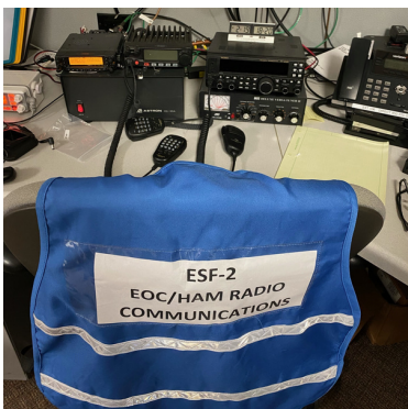
The Ham Radio station at the EOC.
