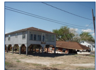
Buildings with foundations that withstand wave action are more likely to survive coastal flooding.
