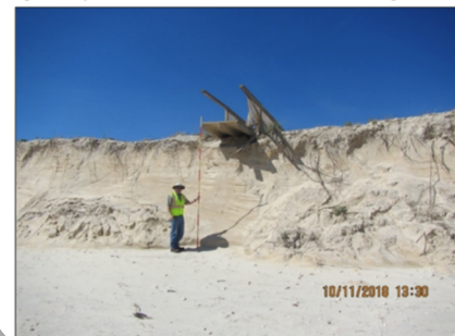
Figure 84. Major dune erosion at R72, St. George Island.
