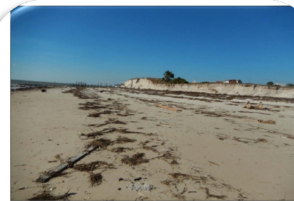
Figure 83. Major beach and dune erosion at Bob Sikes Cut at R52, St. George Island.
